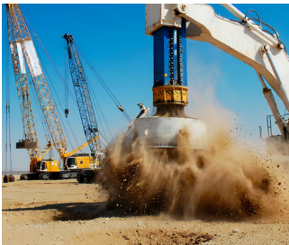
Dynamic Compaction
