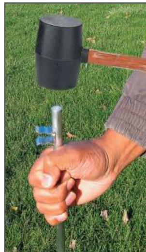
Figure 3. Hard Ground Installation
