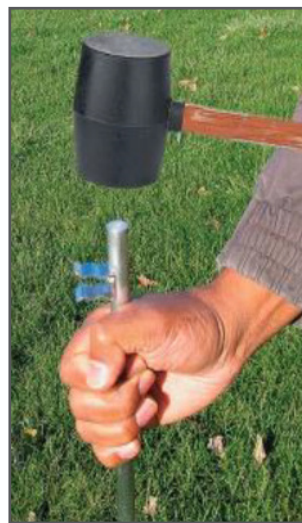
Figure 3. Hard Ground Installation
