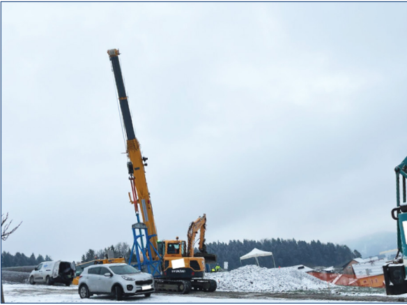
Section C: Pile Testing Škale Viaduct
