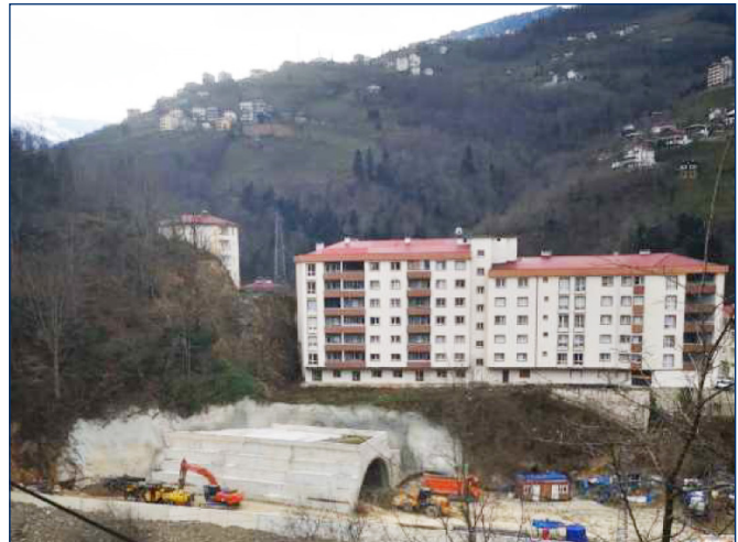
Figure 2 Çaykara Highway Tunnel
