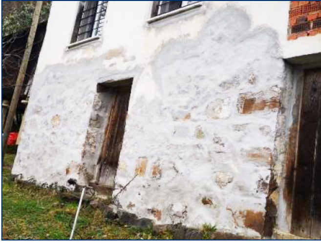
Sensitive historic structures requiring stricter limits for monitoring.
