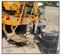
2. Drill the borehole and slide the borehole geophone into place.
